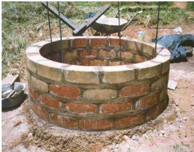
Figure 4 Partially below ground SSB tank under construction (DTU, 2000a)
