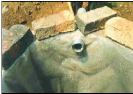
Figure 6 Lining tanks with plastic bags (DTU, 2001b)
