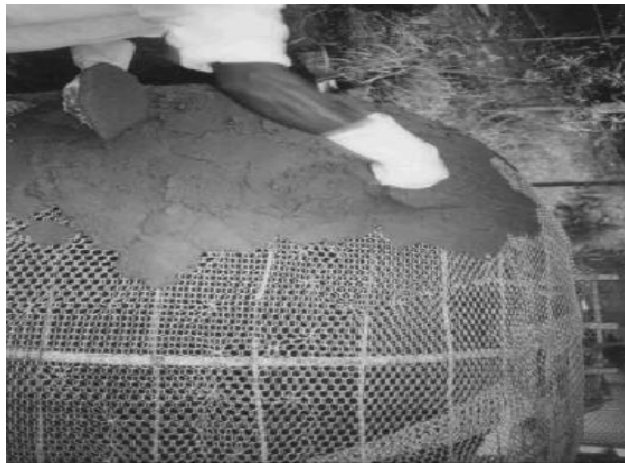
Figure 2 Ferro-cement tank under construction (Turner, 2000)
